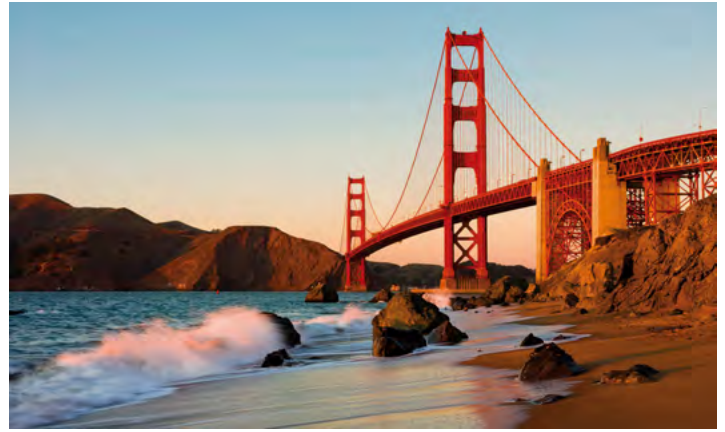
Golden Gate Bridge-San Francisco
